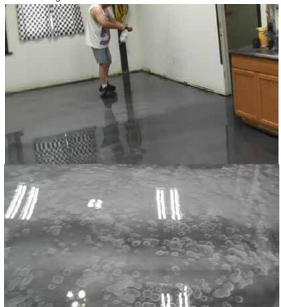
17. The next morning the binder was set up and it was time for the clear. This is pretty straight forward just mix parts A and B and roll out on the floor. Again I used an 18" roller. You're left with one hell of a shiny floor.
